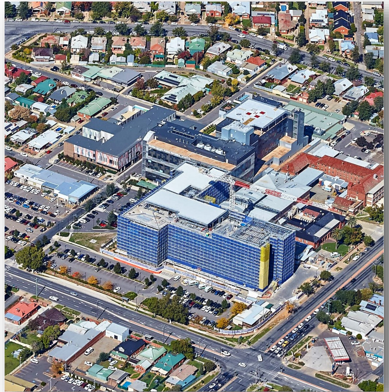
ABOVE: An aerial view of the Wagga Wagga Health Service campus in April 2020. The new Ambulatory Care Building is under construction at the front of the campus.
