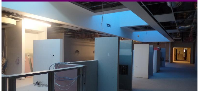
Above: Work is progressing on Stage 1 Recovery First Floor.
