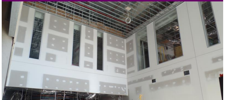
Above: The main Reception area is ready to be painted.
