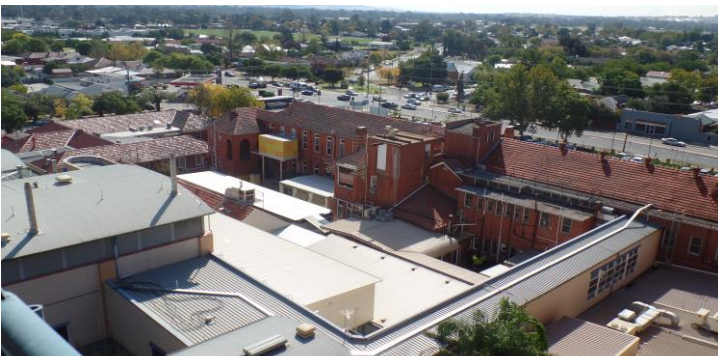
Above: WWBH Back of Campus, Stage 3 Redevelopment.
